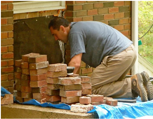
Above, Mike Battistoni applying his masonry skills
